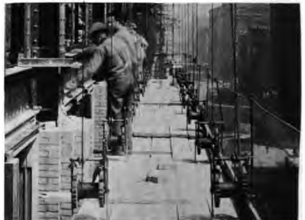
Fig. 3. Approved Scaffold for Building Construction. (Pat.)
